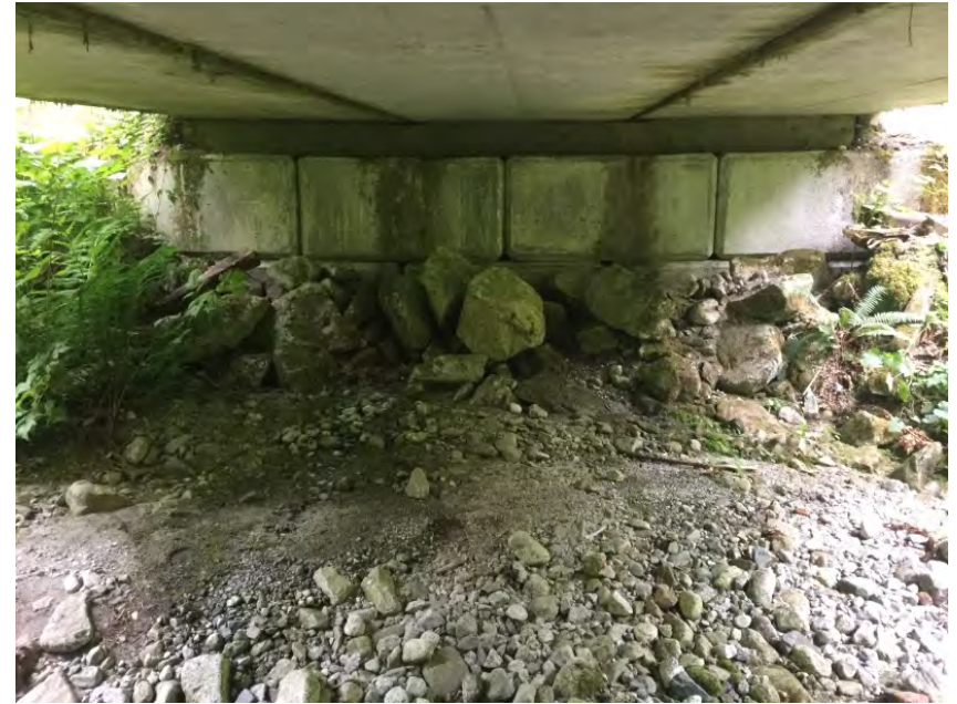
Left Bank Abutment when facing downstream
